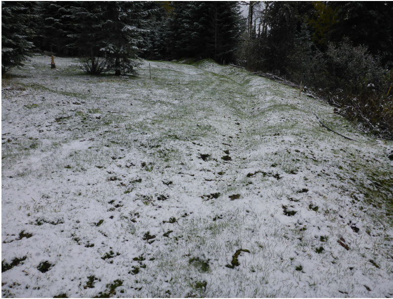
Photograph 3. Condition of ditches – October 8, 2019
